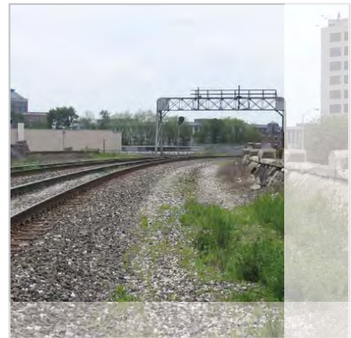
COLLEGE AVE BRIDGE LOOKING SOUTHBOUND
